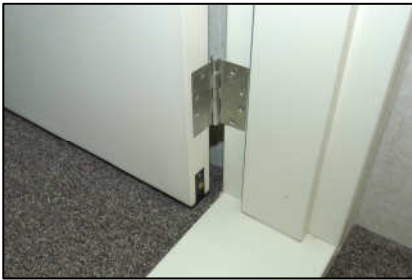
Flush Bottom & Automatic Drop Seal Design to ensure Soundproofing Capability
